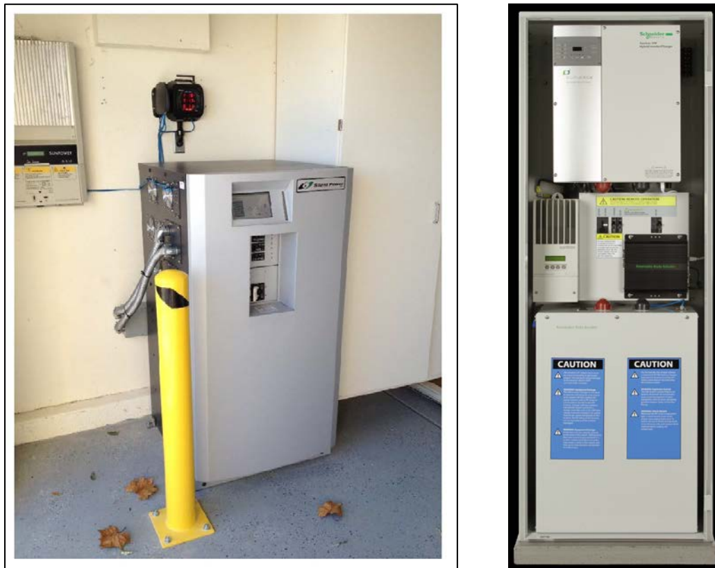
Figure 100. Residential Energy Storage and Energy Management Systems
