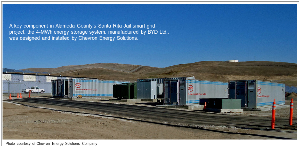
Figure 98. A 2-MW/4-MWh Li-ion Energy Storage System
